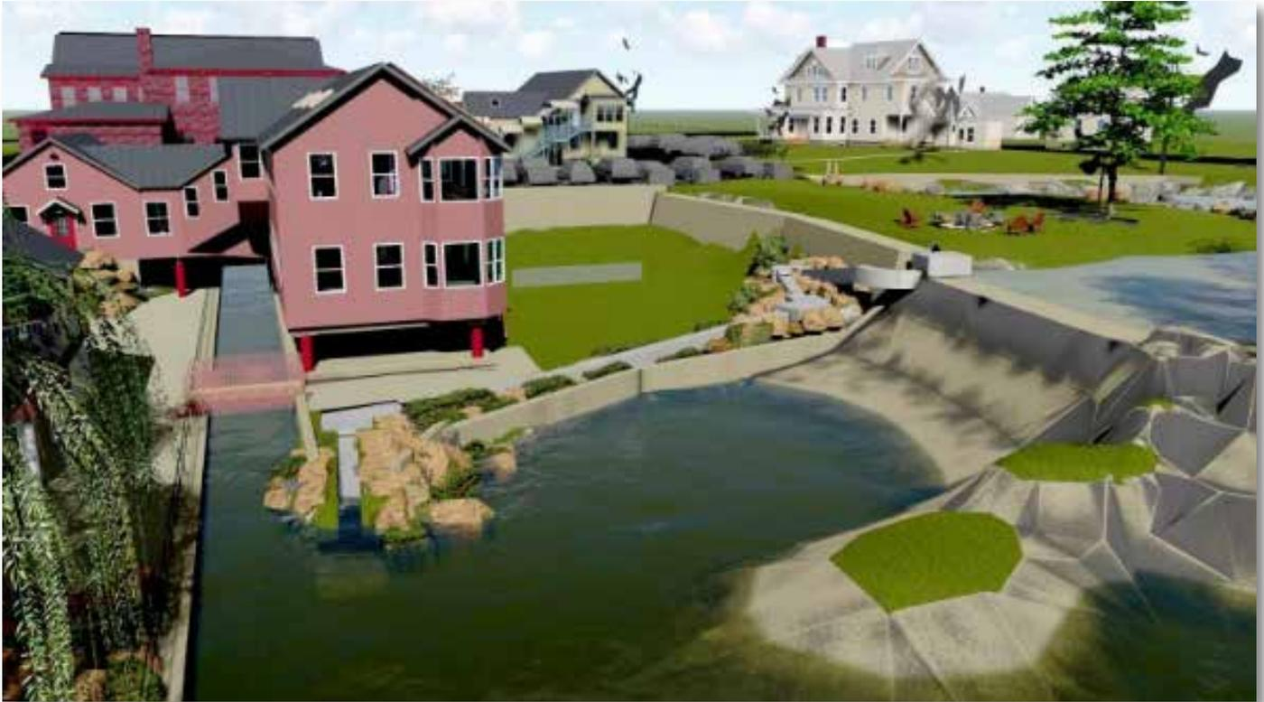
**The fishway behind Centerbrook Architects will allow migratory fish to gradually ascend 18 feet to Mill Pond.** (rendering courtesy of Centerbrook Architects)
