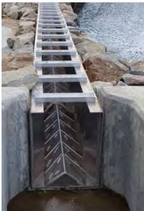
**A close view of the steppass fishway that fish will ascend to reach spawning habitat in Millpond, above the dam behind Centerbrook Architects. The vanes on the bottom and sides slow the velocity of the descending water to allow fish to swim upward. There are several level resting pools along the way.**
